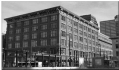
Former Department Store, Denver
